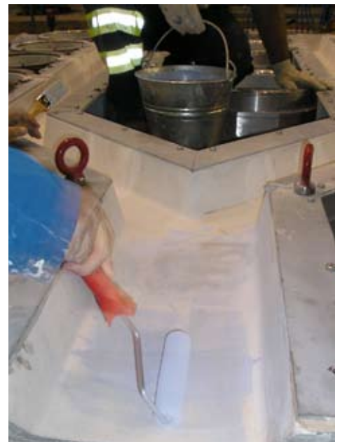
Casting table launder linings at SAPA RC Profiles, Belgium, here being coated with ZYP BN
