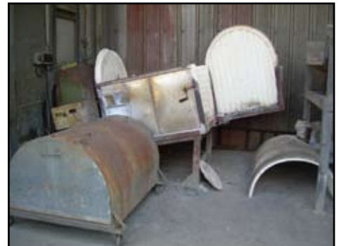
Overview of the MZR without its roof
